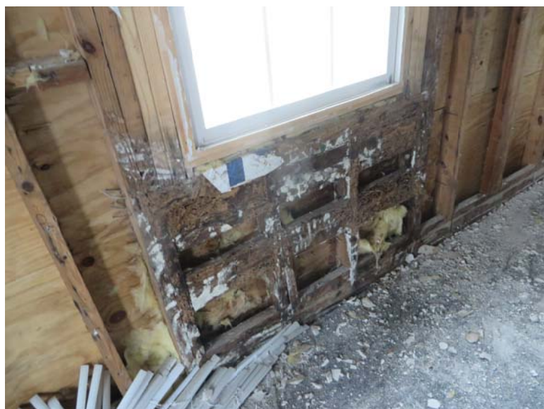
PICTURES OF EXISTING DAMAGED AND DETERIORATED WOOD UNDER WINDOWS. SEE NOTE 3 ABOVE.
