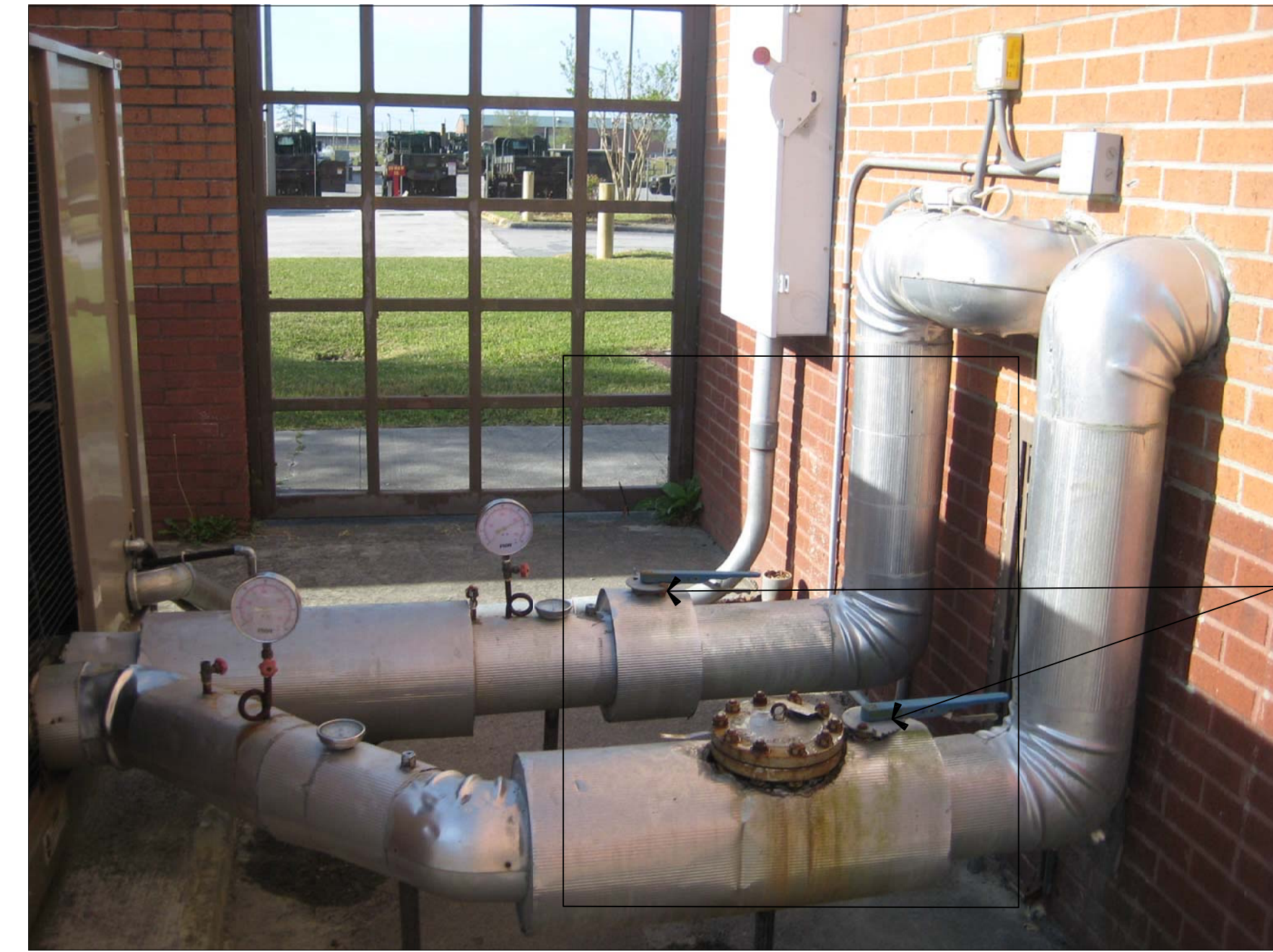
2 REPL. CHWS & CHWR VALVES & INSULATION ON CHILLER W-302 W-302 NO TO SCALE
