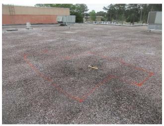
Photo 2 Daylight photo of suspect wet area seen in Photo 1.
