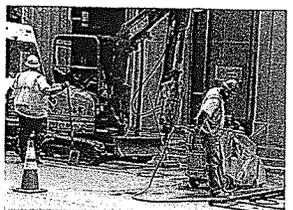
Worker using a walk-behind saw with an integrated water delivery system to cut asphalt roadway. Photo courtesy of OSHA.
