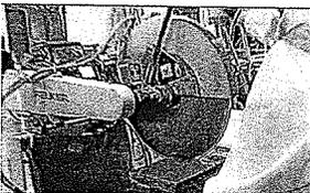
Worker cutting masonry block on a stationary masonry saw equipped with integrated water delivery system that continuously feeds water to the blade. Note water supply hose attached to top of stand around blade.
