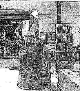
Worker milling granite floor indoors with milling machine and dust collection system (background). Photo courtesy of OSHA.
