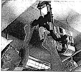
Worker drilling into concrete with a rotary hammer equipped with shroud and dust collection system. Note the shroud around drill bit, silver and black hose, and dust collector are attached conveniently to the drill.
