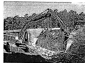
Excavator equipped with an enclosed cab and hoe-ram demolishing a concrete wall. Photo courtesy of CPWR.
