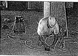
Worker grinding concrete floor with grinder attached to dust collector (background). Photo courtesy of the University of Washington.
