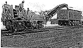
Milling machine milling asphalt road and loading debris into haul truck. U.S. Air Force photo, Beth Holliker. The equipment shown in this picture is for illustrative purposes only and is not intended as an endorsement by OSHA of this company, its products or services.
