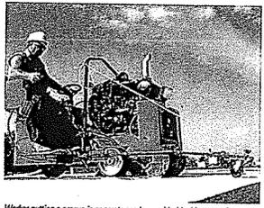
Worker cutting a groove in concrete roadway with drivable saw using integrated water delivery system. Photo courtesy of Hoeghens. The equipment shown in this picture is for illustrative purposes only and is not intended as an endorsement by OSHA of this company, its products or services.
