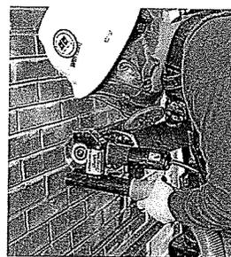
Worker grinding mortar from between bricks with a handheld grinder equipped with a shroud and dust collection system. In addition, worker is using respiratory protection. Photo courtesy of OSHA, International Masonry Institute.
